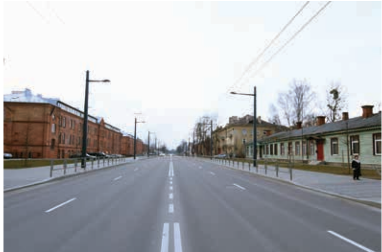
Fig. 3. The main A. Juozapavičius Av. and buildings from Kaunas fortress period – wanted and unwanted in front of each other (photo by D. Babilas, 2016)
